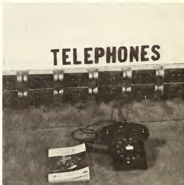
West Point-Pepperell's emergency telephone communications system can be connected to 14 outside trunk lines. The equipment shown in the picture is installed in the civil defense control room at the company's Langdale Mill.
